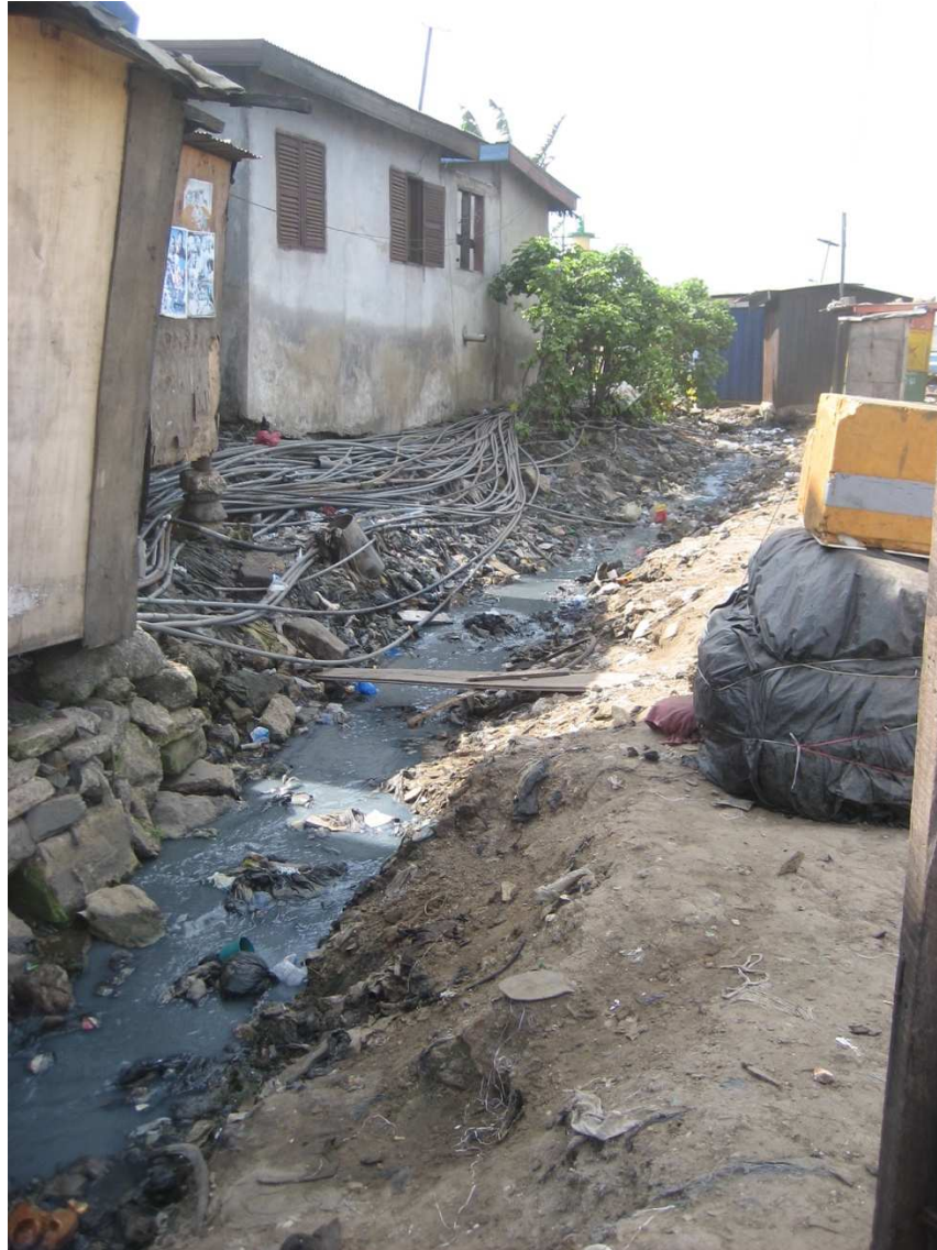
Figure 19. Self-installed water network pipes “spaghetti pipes” running along the ground near drainage flow in Agboghloshie, Accra. This situation is representative of many neighborhoods in Accra Metro (Photo credit: Paul Cottavoz).
